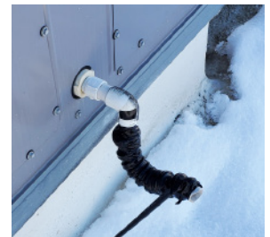
SpeedTrace heating cable wrapped around an outdoor pipe
