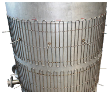
Mineral Insulated (MI) Heating Cable
