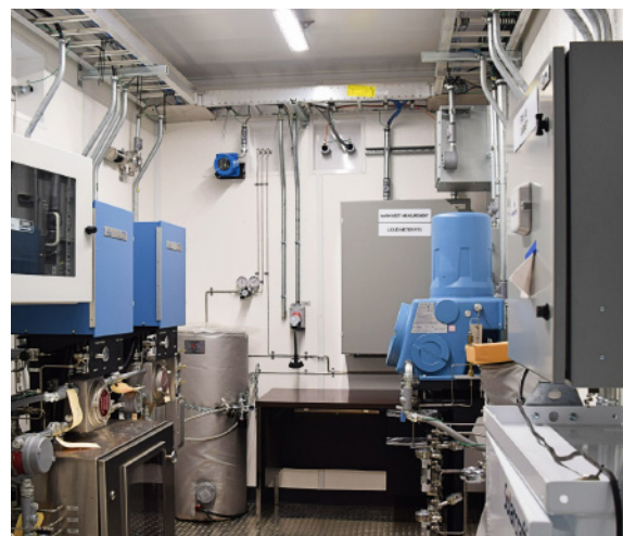
Analyzer Shelter with Gas Cylinder Warmer in use
