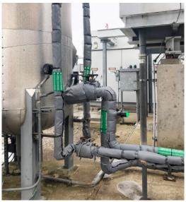
reusable, suitable for use outdoors, and constructed of ultra-durable PTFE outer cloth material with energy-efficient 1 in (25 mm) thick fiberglass insulation. Access to the piping for maintenance is very simple. As an added bonus, the most common insulator sizes and shapes are in stock for quick delivery and BriskHeat is able to design customs for most shapes and sizes to fit nearly any application.
