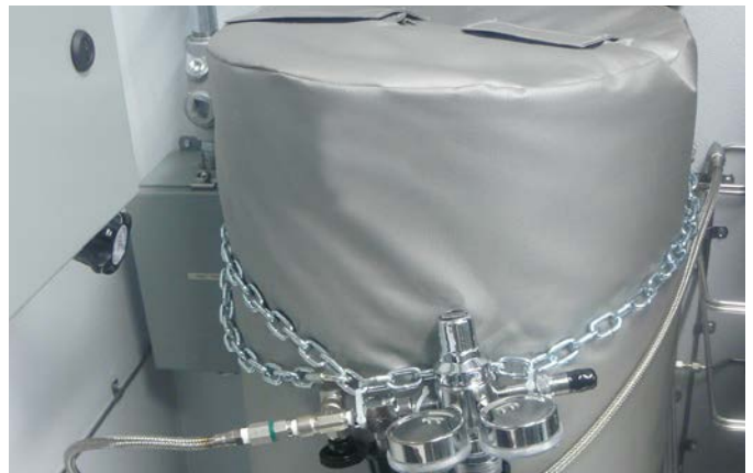
Hazardous-area rated gas cylinder warmer
