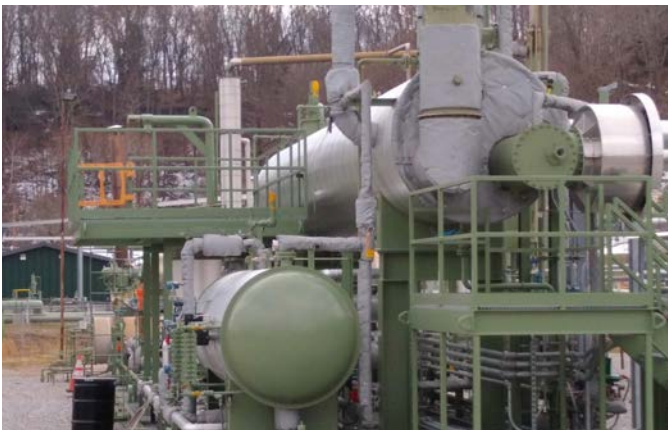
Removable insulators and heating cable installed at compressor station
