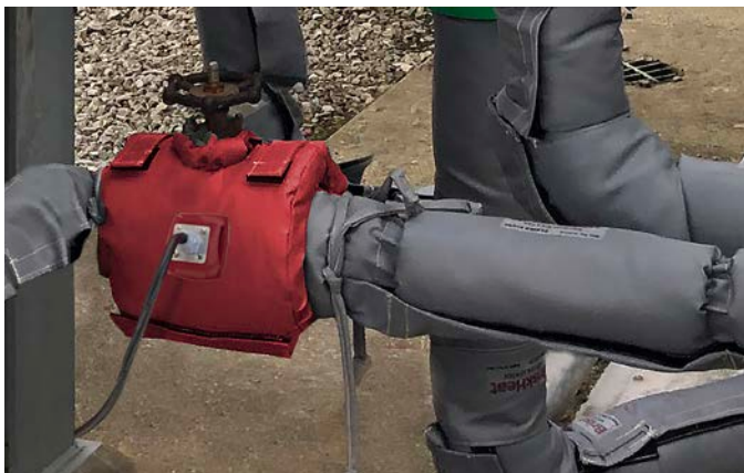
Cloth heating jacket installed on valve for freeze protection
