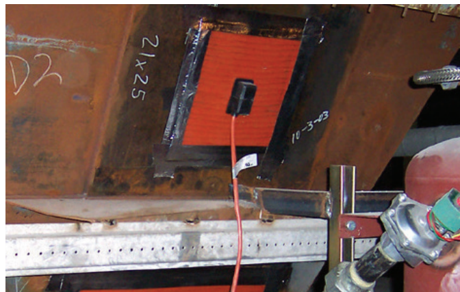
Silicone rubber heating blankets installed on a vessel
