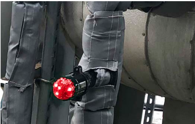
Installation of monitor light, heat trace, and removable insulators on pipe system
