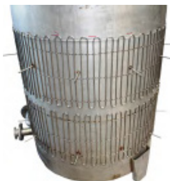
MI Mineral Insulated Heating Cable
