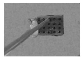
5. Install heating cable. Use pliers to close clamps, but do not crush the heating cable.
