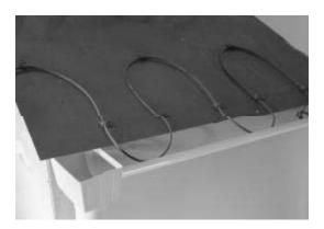
3. Orient the clip as needed. Attach clip to roof using a nail or a screw.
