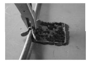
2. Apply sealant, appropriate for your roof, to back side of clip where nail or screw will be used.
