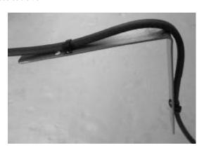
3. The SLCBL-RDOWN1should be centered on the edge of the downspout to prevent mechanical damage and to support the heating cable.
