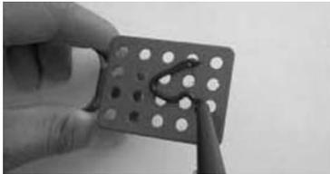
3. Orient the clip as needed on the roof. Place the roof clip on the roof where the roof is marked. Press down on the clip so that the adhesive flows through the holes. The cable insertion clamp should be vertical on the roof. Attach the clip to the roof using a nail or a screw.
