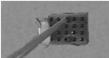
4. Apply sealant on top of the nail or screw heads.
