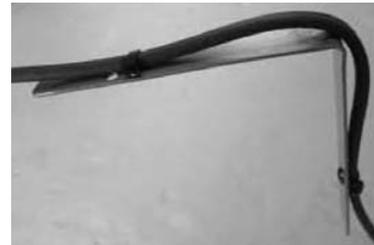
3. **Note:** If installing the cable in a gutter at the end of a run, do not allow the end of the heating cable to stick out in the air at the end of the downspout. Instead loop the cable back up the downspout a minimum of 1 ft(30cm) and connect with a cable tie as shown.
