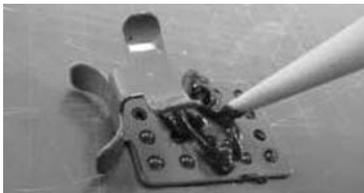
5. Allow the RTV adhesive to cure and dry before installing the cable. Refer to the RTV adhesive instructions for the cure time of the adhesive used.
