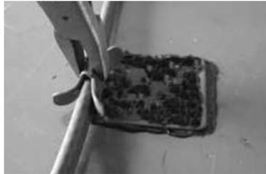
8. Run the cable from the starting point and use a roof clip to connect the cable to the edge of the roof.
