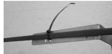
2. Tighten the cable ties to secure the cable. Trim off the excess ends of the ties. Do NOT cut the heating cable.
